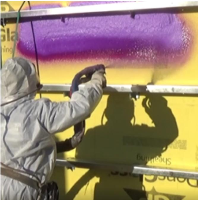
1. Apply spray foam directly to sheathing. Application will need to occur within the recommended temperature range.
