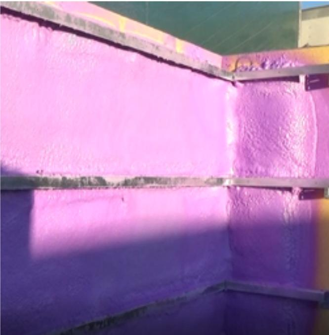
11. With the insulation installed and the girts cleaned, you now have a continuously insulated exterior wall ready to be cladded.
