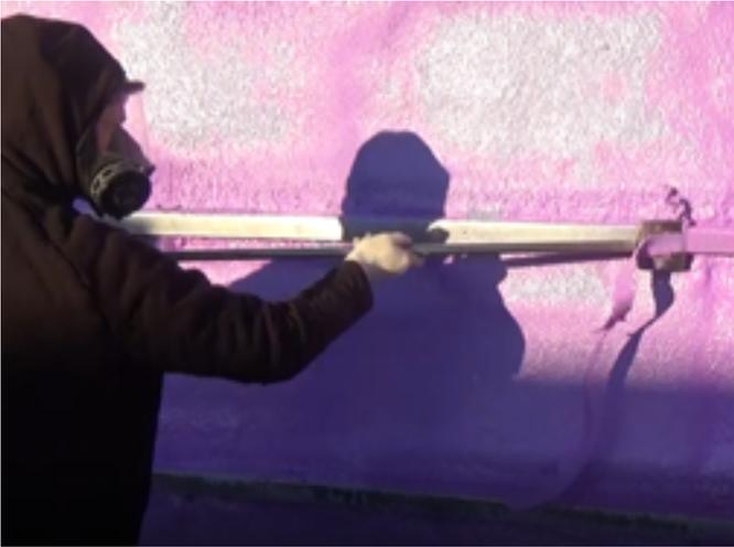
8. Once spray foam is installed and allowed to cool, scrape girts to remove overspray, so it does not interfere with cladding installation.
