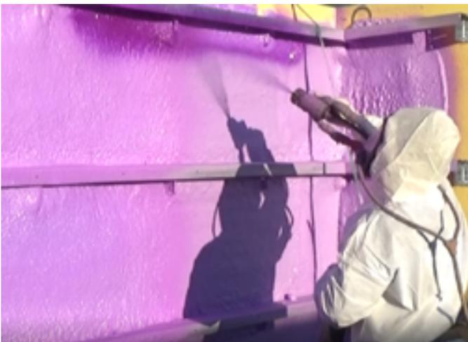
6. Multiple passes may be required for application in excess of 50mm or 2in. This may vary depending on the product used. If this is required, ensure the first pass is allowed to cool before applying the second pass. Refer to product details and recommendations before installation.
