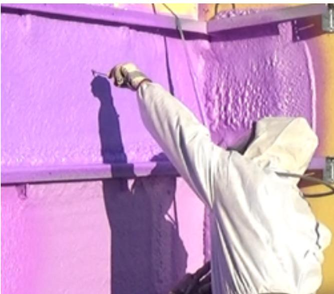
7. Check insulation depth throughout insulation application to ensure desired depth is achieved.
