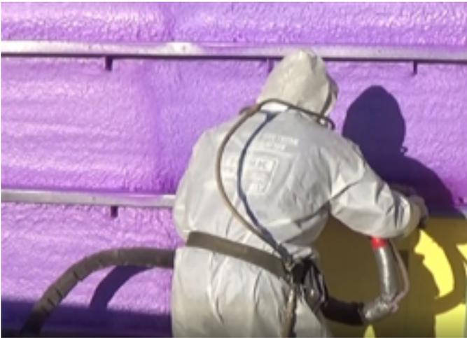
4. Space between the girt and the sheathing will need to be minimum 1/2" more than the desired insulation depth to accommodate variation in spray foam thickness and over spray.
