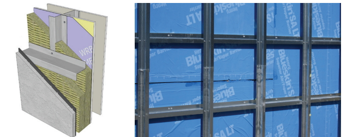
Crossing Z-girt assembly consisting of horizontal and vertical Z-girts attached at crossing points.
