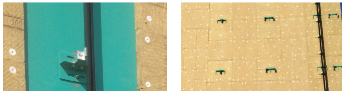
Example of heavy-duty engineered anchor consisting of large welded steel plates and vertical rail system.
