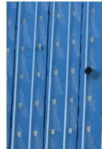
Intermittent galvanized steel clips with vertical girts.
