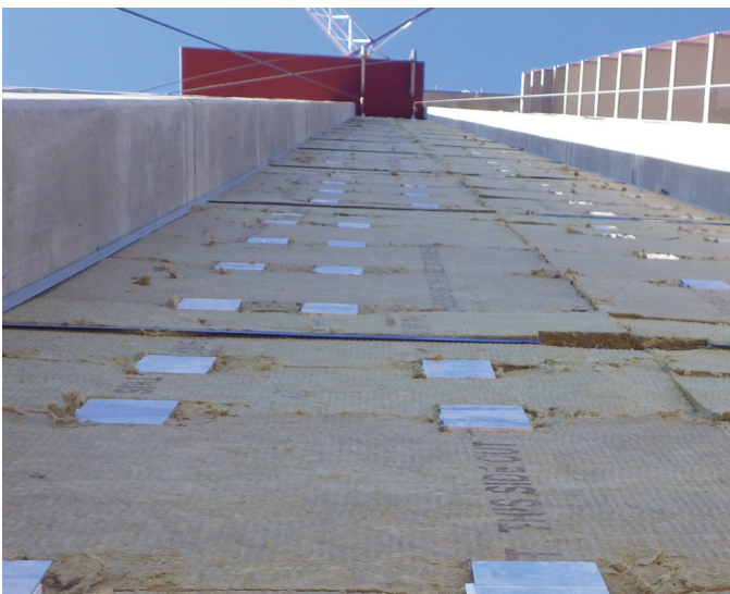
Example of insulation retained by intermittent cladding support clips behind metal panels. The metal panel support structure overtop will further retain the insulation in the assembly here.
