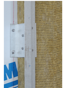
Generic adjustable back to back L-angle clips.
