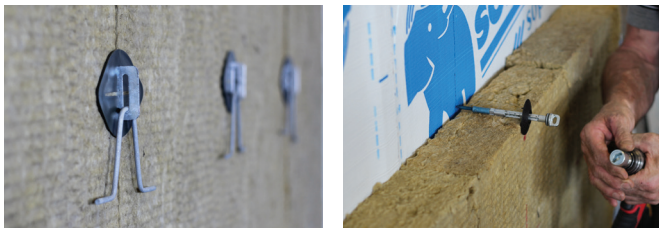
Examples of masonry ties installed through ROXUL CAVITYROCK® insulation.
