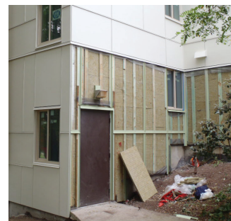
Long screws through vertical wood strapping and rigid ROXUL COMFORTBOARD™ insulation on a multi-family residential project.
