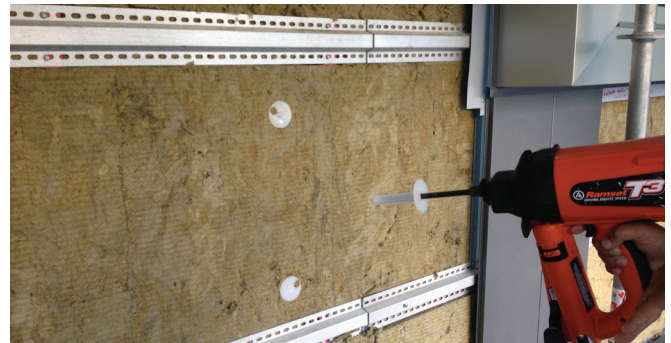
Example of plastic fuel-cell actuated insulation fasteners installed after insulation and girt system is installed to retain the insulation.
