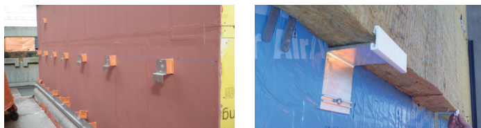
Examples of thermally improved discrete cladding supports for composite metal panels.
