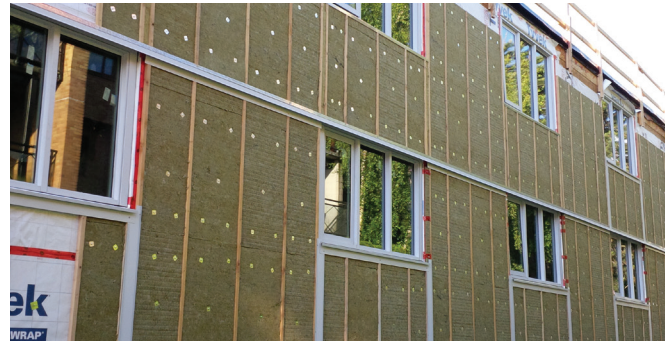
Example of insulation retained by mechanically attached impaling pins between vertical wood framing (adhesive stick-pins are not considered a long-term support strategy).
